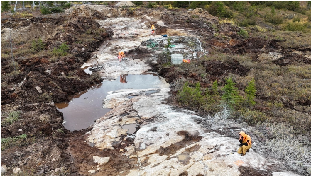
Photo 4 - Lithos South. Stripping in progress enlarging already known outcropping spodumene pegmatite (view looking north).
