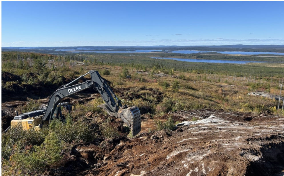
Photo 1 - Mechanical stripping uncovering near-surface spodumene pegmatite. Yo-Yo sector.
